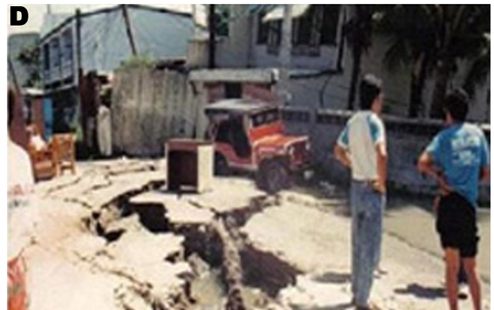
Figure 10. Manila Bay reclamations can be severely damaged by distant earthquakes. A, In 1968 a Magnitude Ms 7.3 earthquake in Casiguran, Quezon caused severe damage in Manila, 225 km away, and the 1990 Ms8 earthquake, with its epicenter in Rizal, Nueva Ecija caused massive destruction in Dagupan City, 10 km away ( B,C, and D ). B, Truck that sank into liquefied ground; C, Tilted building; and D, fissures and lateral spreading.
