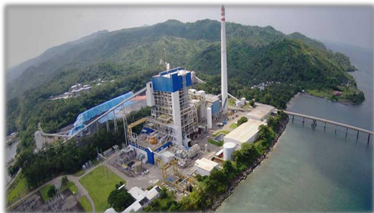
Figure 18: The 1 st Supercritical Coal-Fired Power Plant in the Philippines by San Buenaventura Power Ltd. Co., with a capacity of 550 MW located in Mauban, Quezon (Cinco, 2020).
